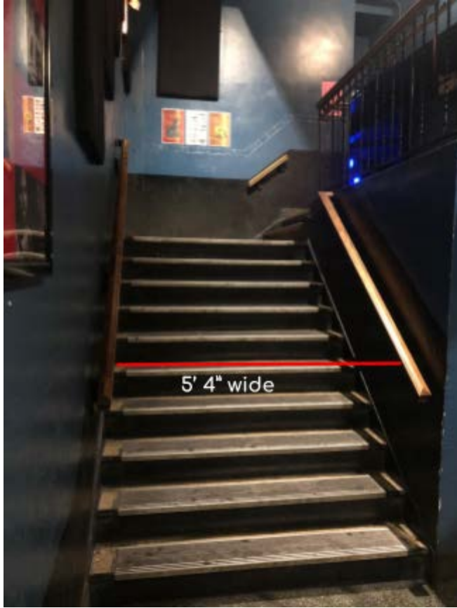
10 STAIRS UP TO SMALL LANDING
