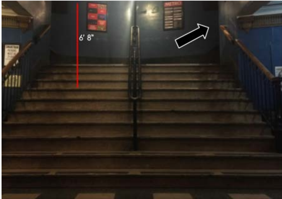
12' WIDE STAIRCASE WITH CENTER RAIL CEILING CLEARANCE AT HIGHEST STAIR (7TH STEP) IS 6' 8"
