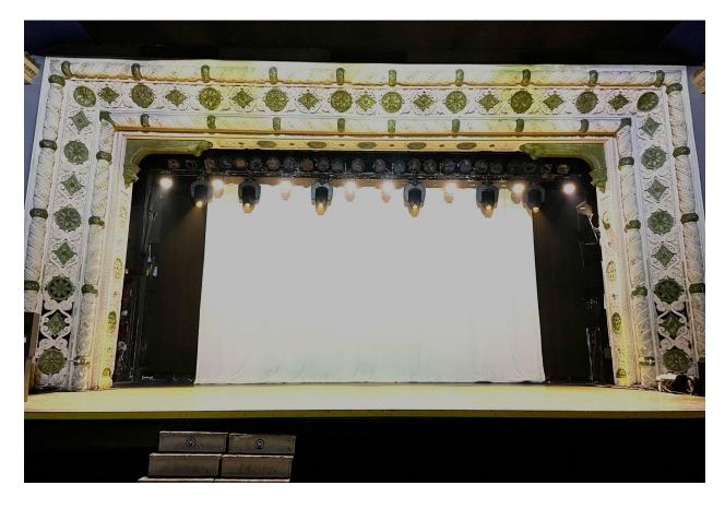
24' x 20' WHITE CURTAIN Hung from catwalk with clamps - LX truss does not raise / lower
